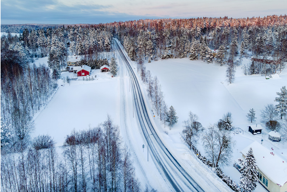
Aerial view of a road in the winter snow forest in Lapland, Finland.
