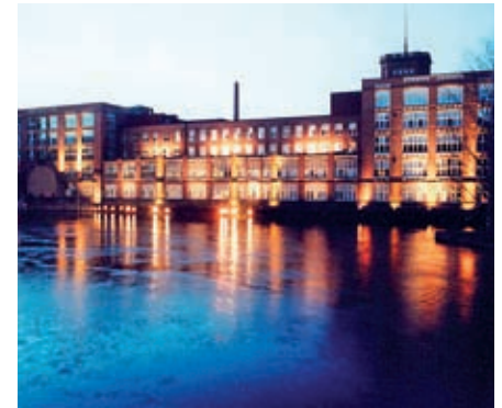
Figure 3: A view of the Tampella building (Source: picture by Mariangela Lavanga)
